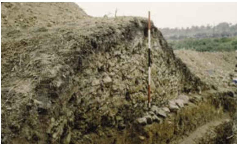
Professor Anne Robertson's section through the Antonine Wall at Tentfield Plantation, east of Rough Castle, in 1959 reveals many layers of turf work erected on a stone base. These turves provide valuable information on the nature of the vegetation at the time the Romans started to build the Wall.
